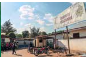
Bangui Pediatric Hospital Complex Central African Republic
