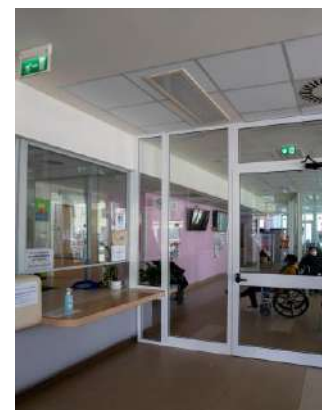
Glass wall and door installed to separate patients
