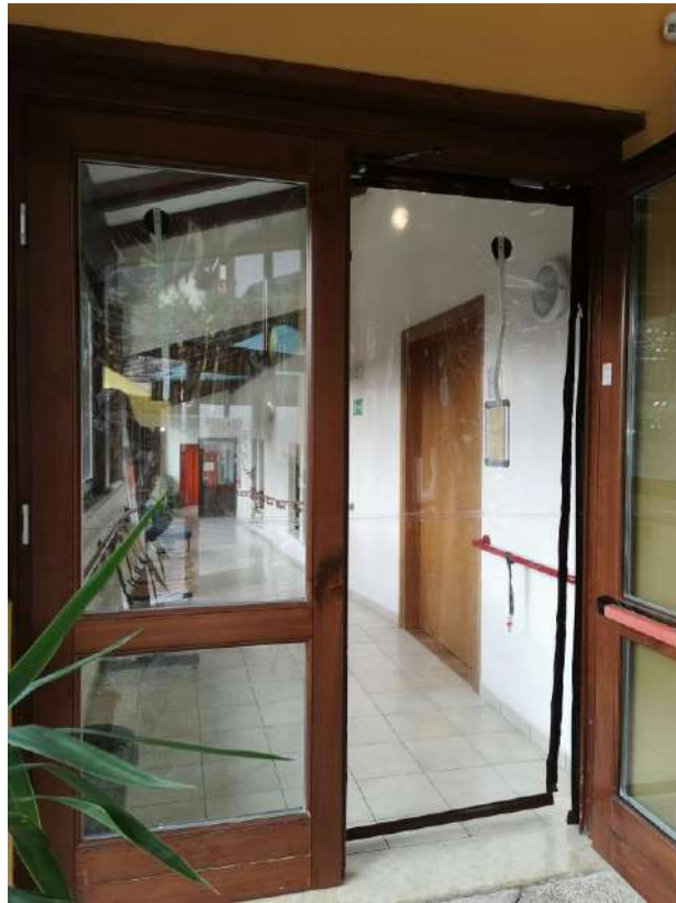
The automated door used as a separate entry for personnel
